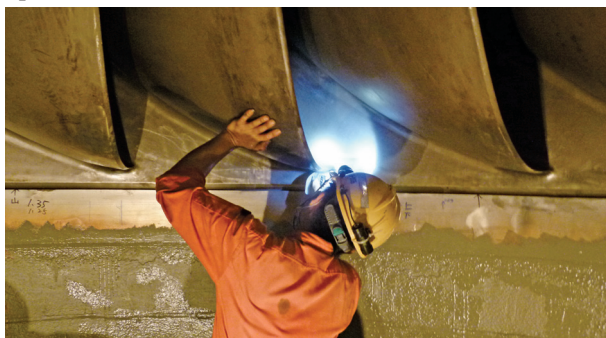
▲ Feitsui Power plant repairing (internal turbine inspection)
